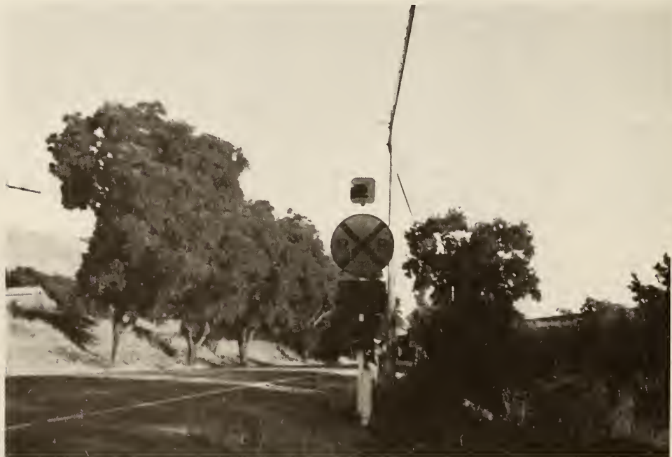
Figure 41 Activated Advance Warning Device (Southern Pacific Crossing)
